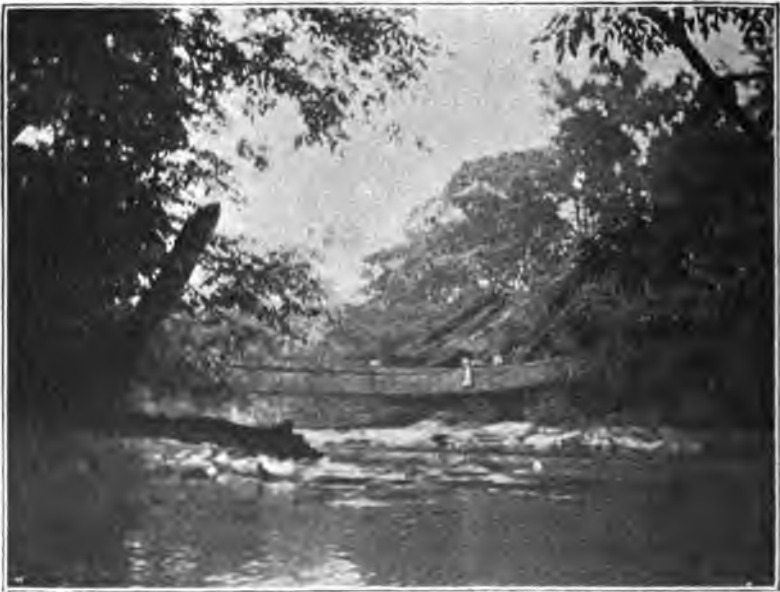
HAMMOCK BRIDGE OVER SELI RIVER.
