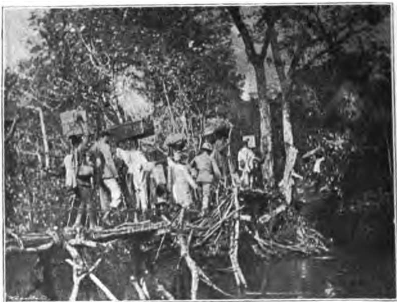
CROSSING TRESTLE BRIDGE.
