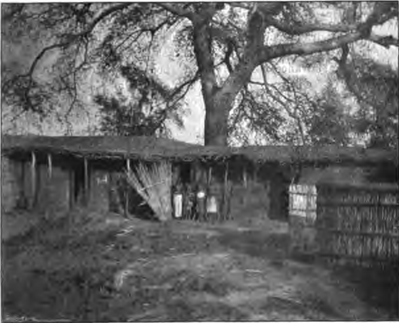
WALL OF KAMBWIRE'S KRAAL, FROM INSIDE.
